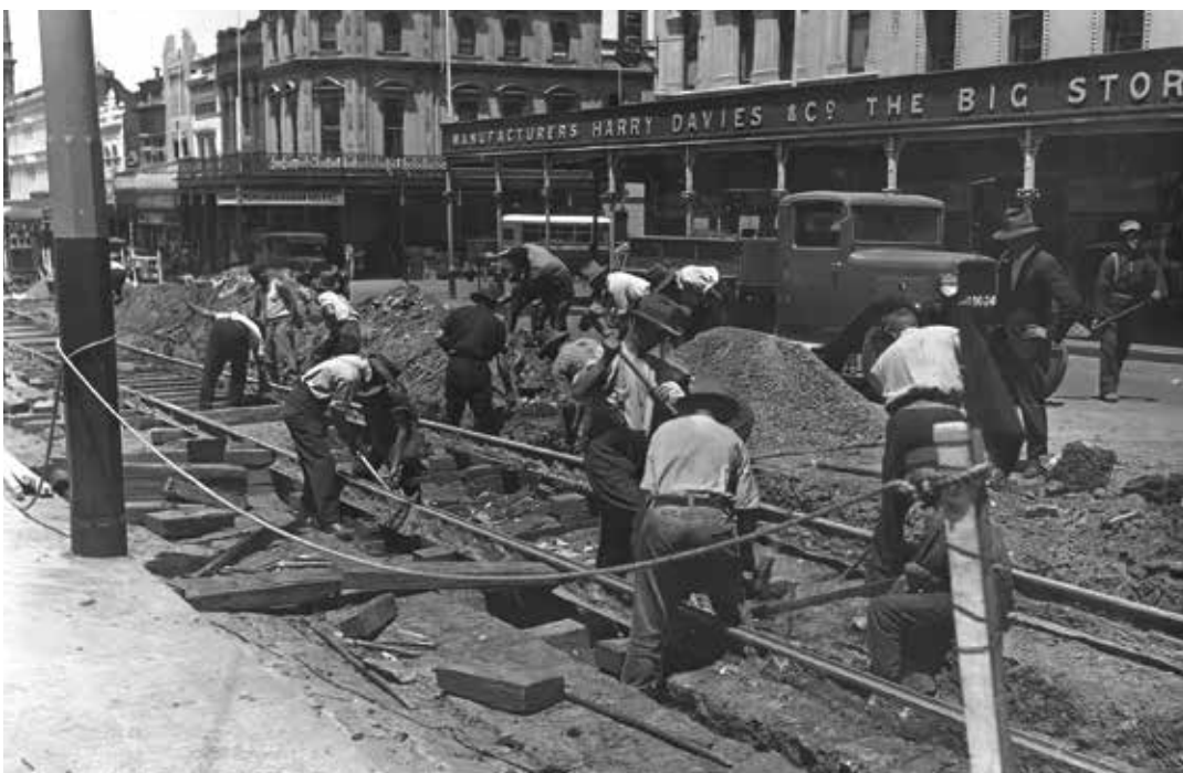
The uncropped front cover image showing the tramways rehabilitation works conducted by the SEC in 1934. The work provided much needed employment for many Ballarat men during the worst of the depression.
