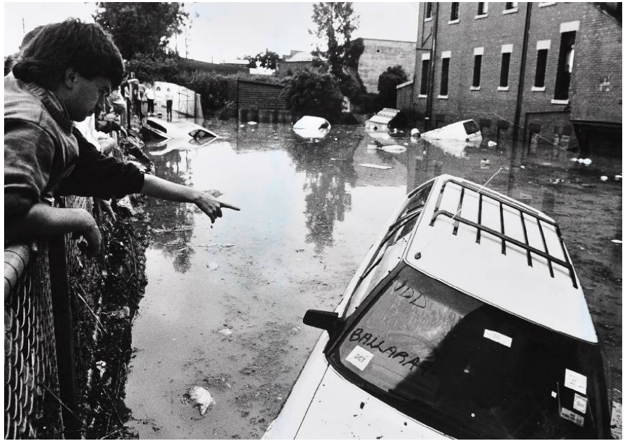
Cars bob in the floodwater behind SF Motors in Lydiard St Nth. December 10 1988.
